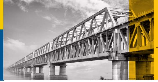
Rail cum road Bridge over river Ganga with spans as long as 123 M in length involving 36000 Ton of steel fabrication and erection
